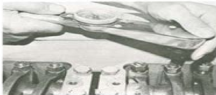
Fig. 14-101, DN114063. Adjusting injector plunger
