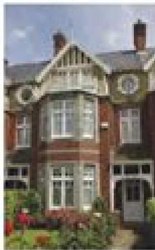
1.29 During the Victorian period, there was a new for contrasting materials such as different materials and more varied window patterns, a new pattern from the Arts and Crafts movement.
